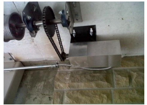
Installed GearMotor with GDI's mounting bracket
